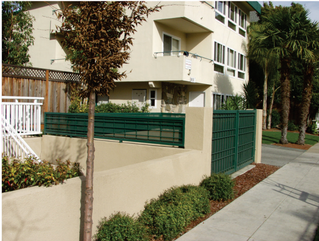
TRANSFORMER ENCLOSURE EXAMPLE (San Mateo Metropolitan Apartments)
